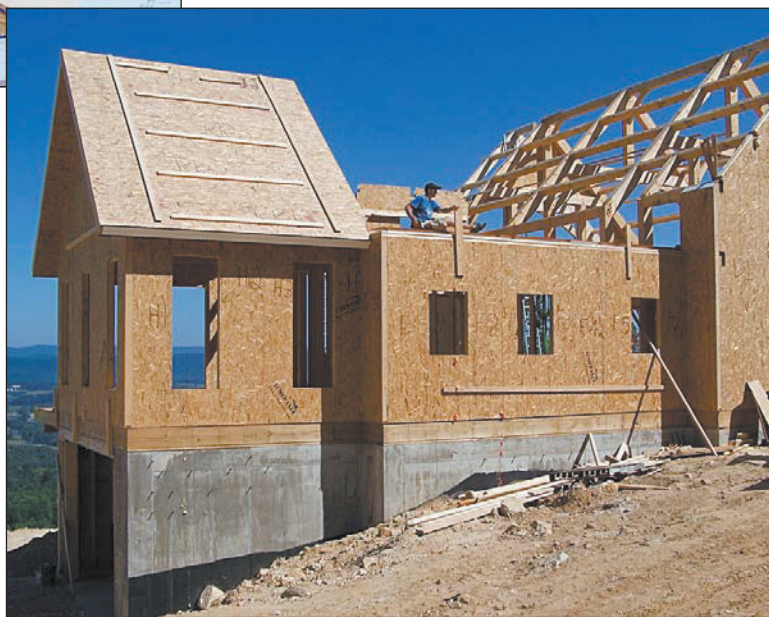
Acme (America's Cleaner More Efficient) Panel company is owned by Joe Fortier of Taylor Hollow Construction. The panels (top right) are energy-efficient, strong and have reduced greenhouse gas emissions. They are used in commercial and residential (left) construction.
